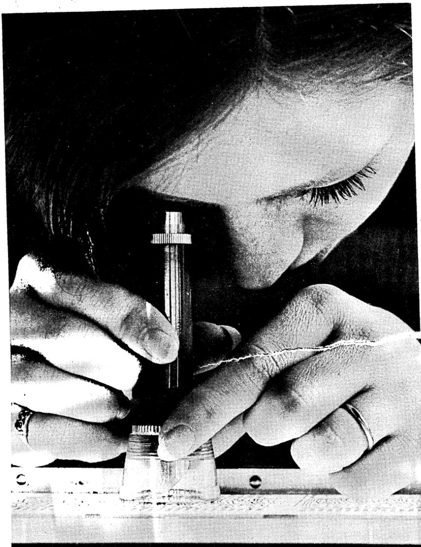
All DEC modules are exhaustively inspected and tested, both visually and electronically. A typical module undergoes a printed circuit board inspection procedure that consists of over 70 individual steps.
